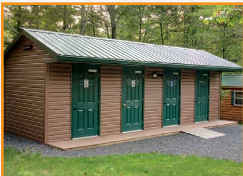
13x28 Campground Bathhouse
