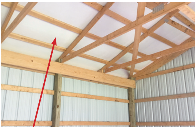
Double Bubble (Condensation Barrier) A Popular Roof Option. Also a Great Idea on the Walls.
