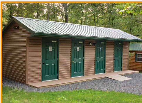
13x28 Campground Bathhouse
