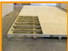
Pressure-Treated Skids and Floor Joists
